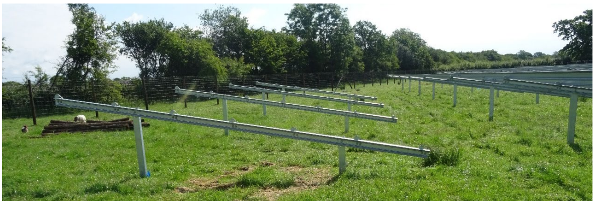
Photograph 15.5: Framework Posts Installed (taken at Bentham Farm, Purton 2015)
