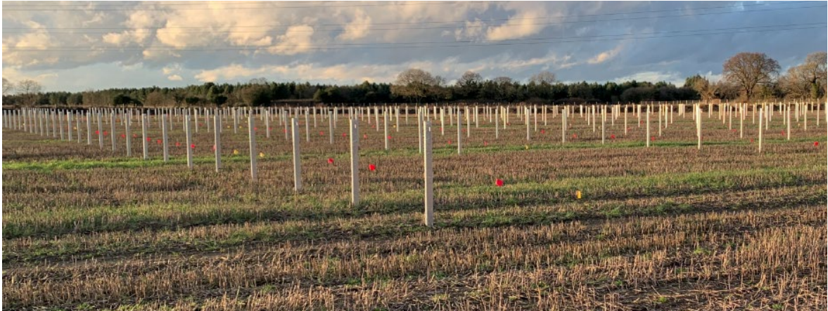
Photo 15.6: Framework Posts being Installed (taken at Tiln Farm, Retford, in January 2023)
