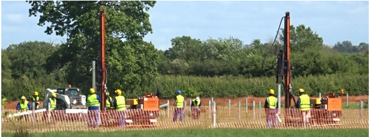
Photograph 15.4: Framework Posts being Installed
