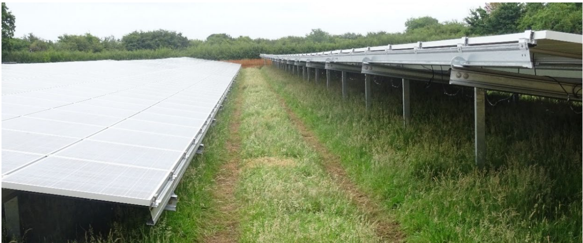
Photograph 15.7: After Solar PV Panels Bolted-on (Bentham Farm, Purton)
